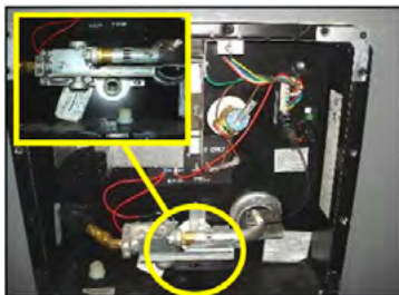
Fig 1: Water heater drain plug
